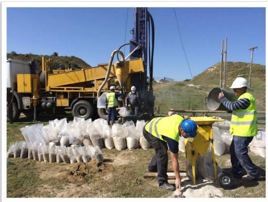
Figure 1: Drill hole MAC-RC-014 in progress with Plymouth personnel sampling in the foreground with bags in the background located at recently completed drill holes.
