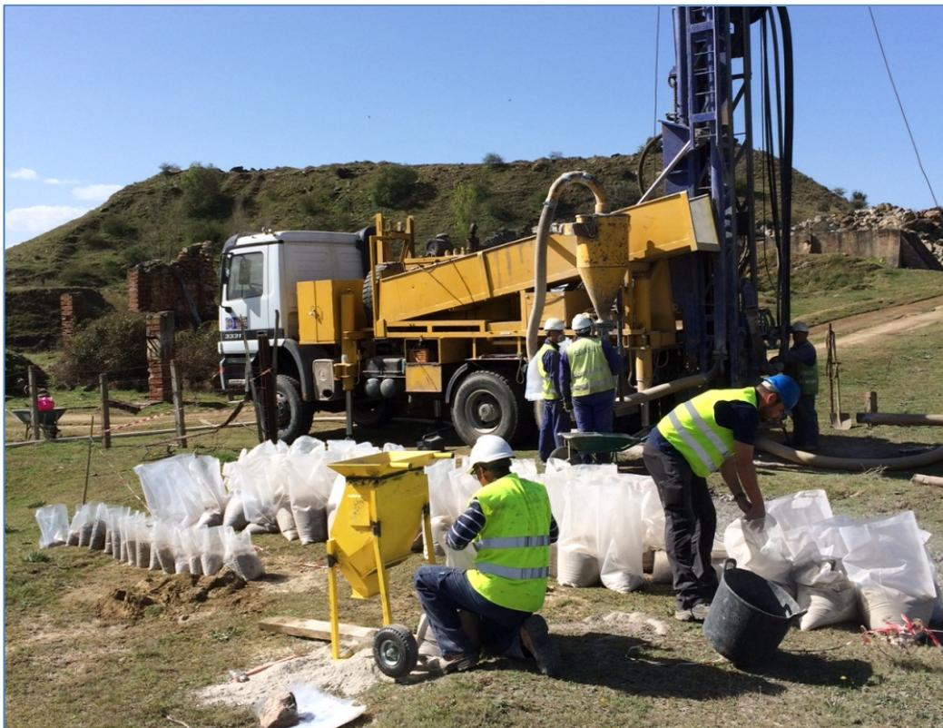
Figure 2: Drilling underway at Minas Alegria (old process facility buildings visible in background) with sampling underway in foreground. MAC-RC014
